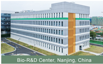
Bio-R&D Center, Nanjing, China
